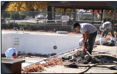
Butler Pool being repaired last November
