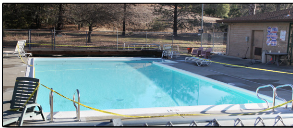
Butler Pool with completed repair work in January
