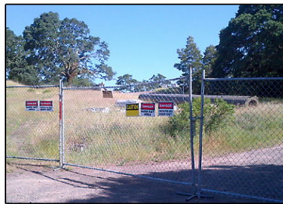
Cell tower under construction [photos by JJ Fernandez]
