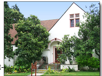
New Employee Orientation takes place at McDougall
